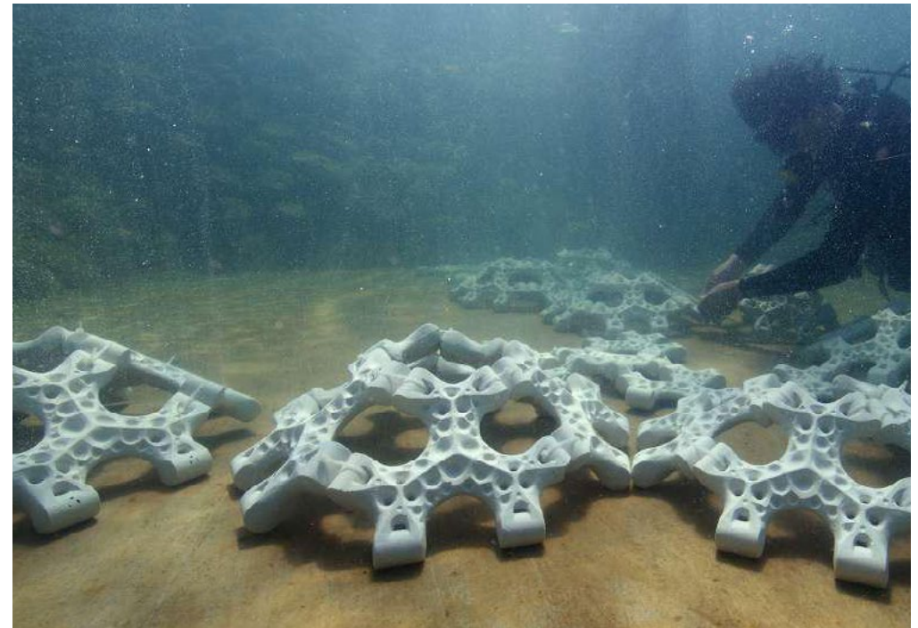
Gilberto Esparza installing elements designed to help growth of corals
