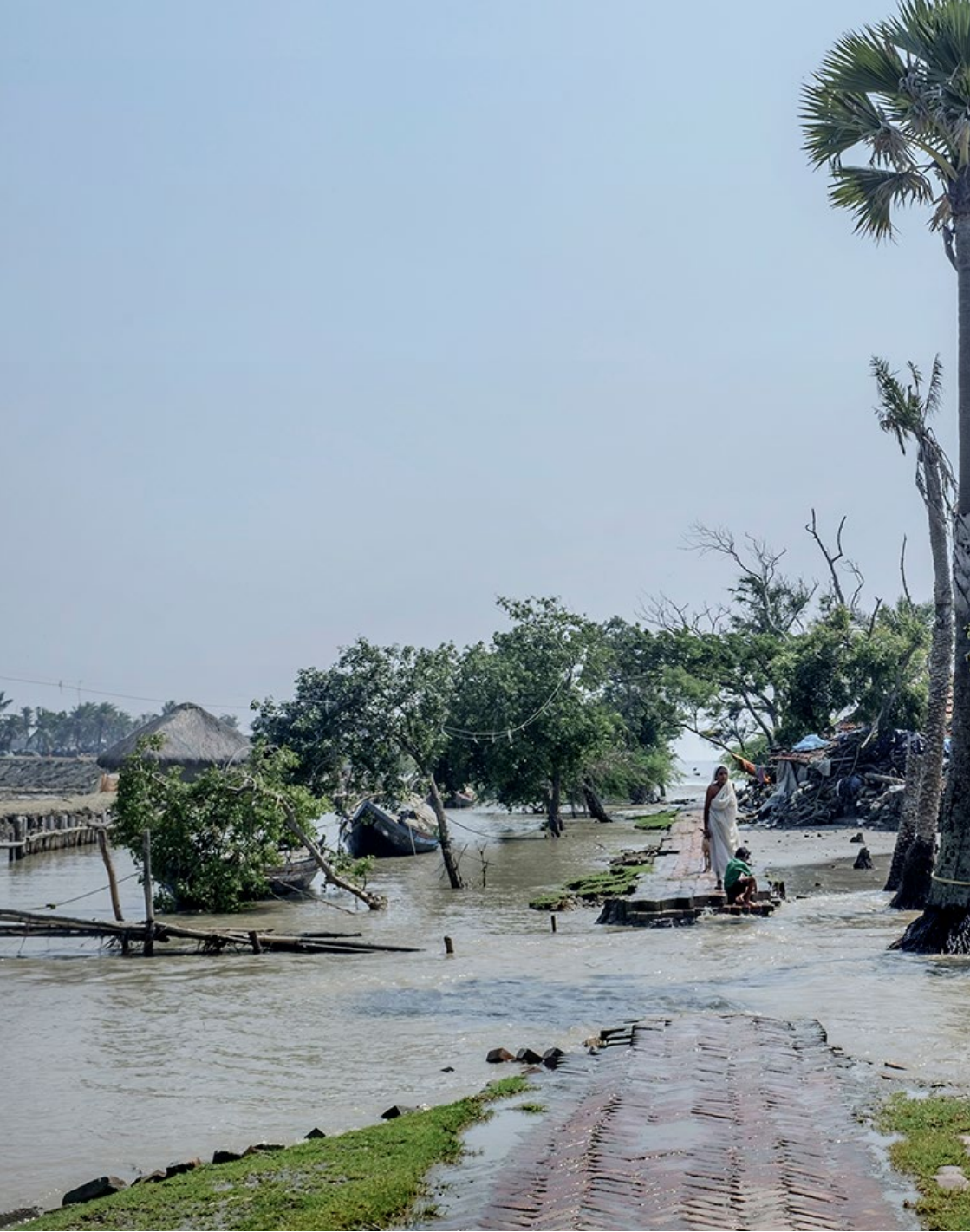
Tidal surges during monsoons effectively cut off certain zones from land. Sagar Island, India. © Arko Datto
