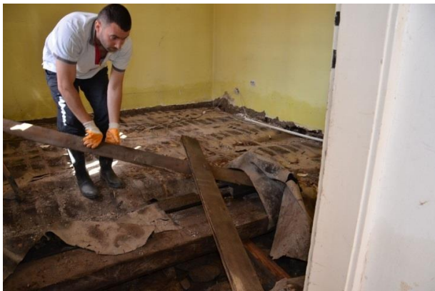
Work begins on replacing the floors
