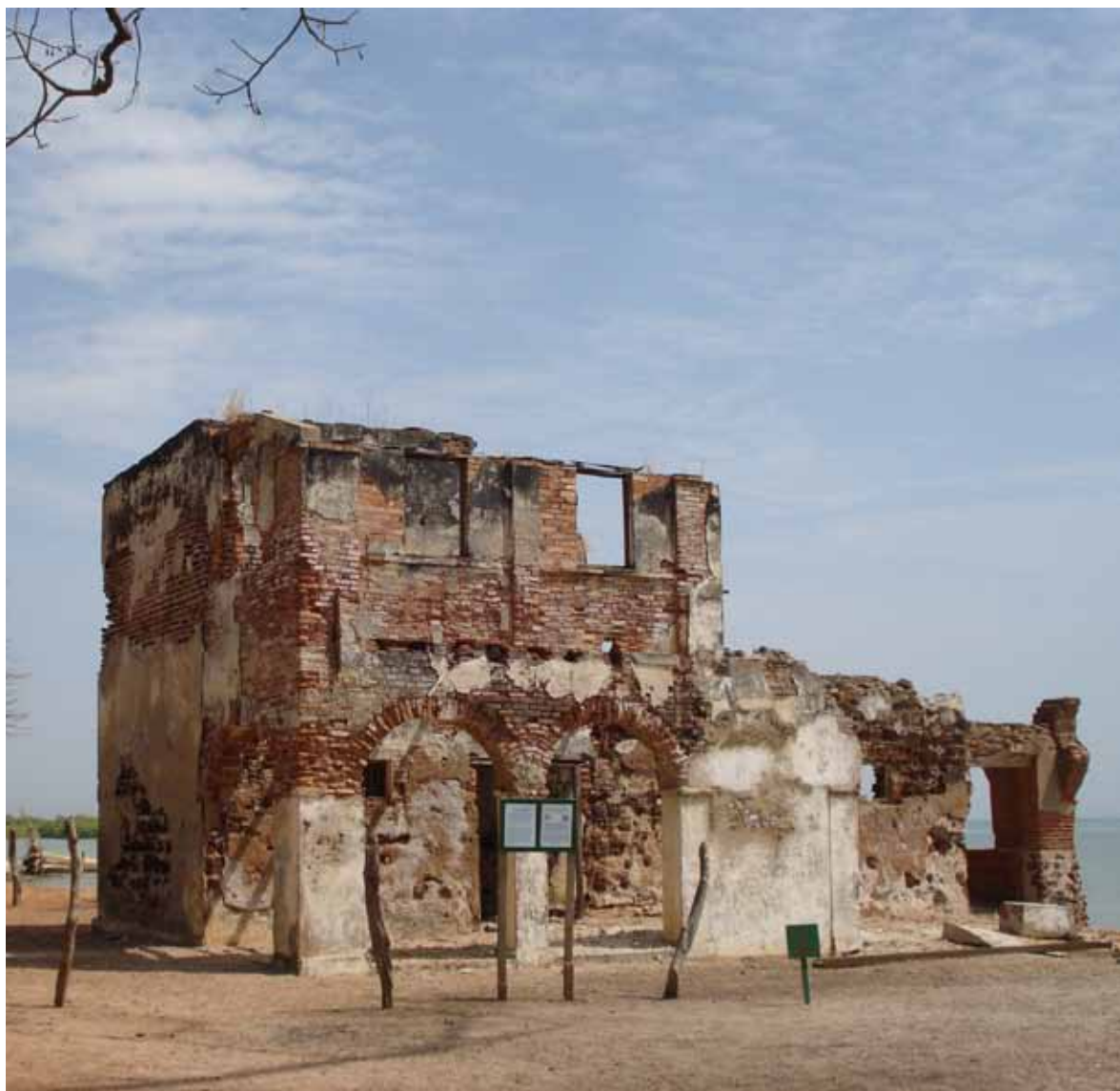
The CFAO Building in Gambia that was restored with support of the CER programme
