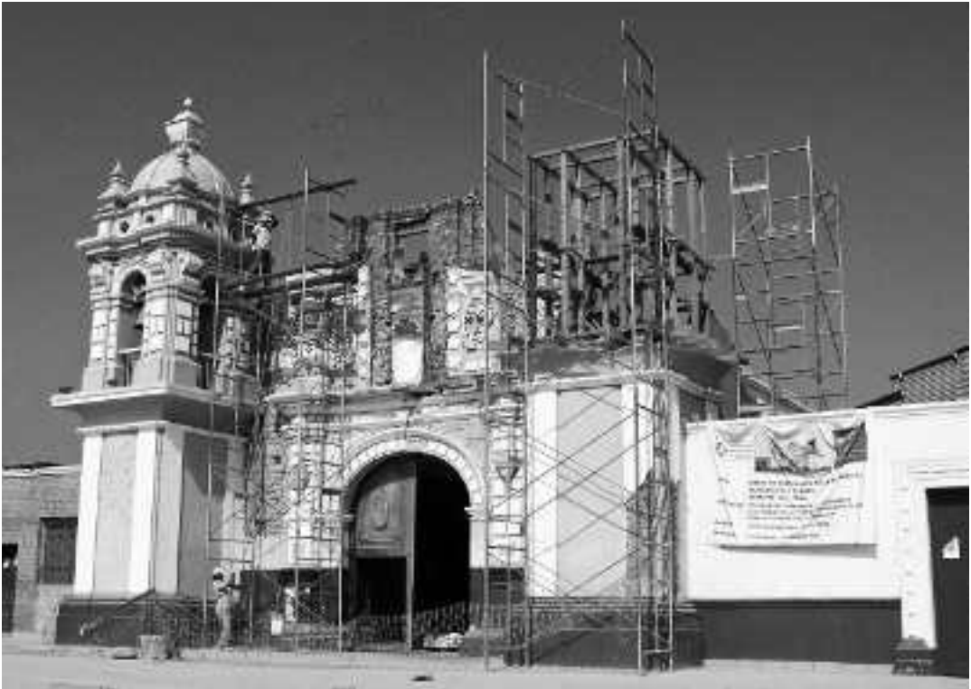
The Church of El Carmen in Ica, Peru, surrounded by scaffolding.
