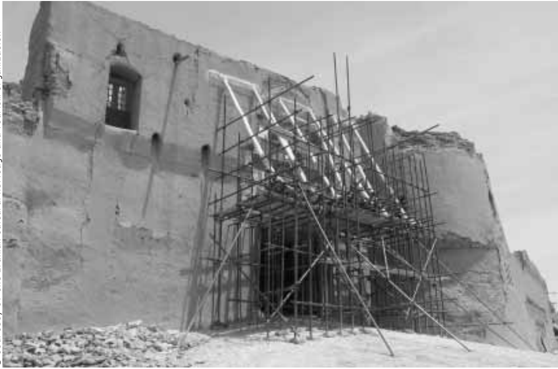
Restoration of the citadel in Bam, Iran.
