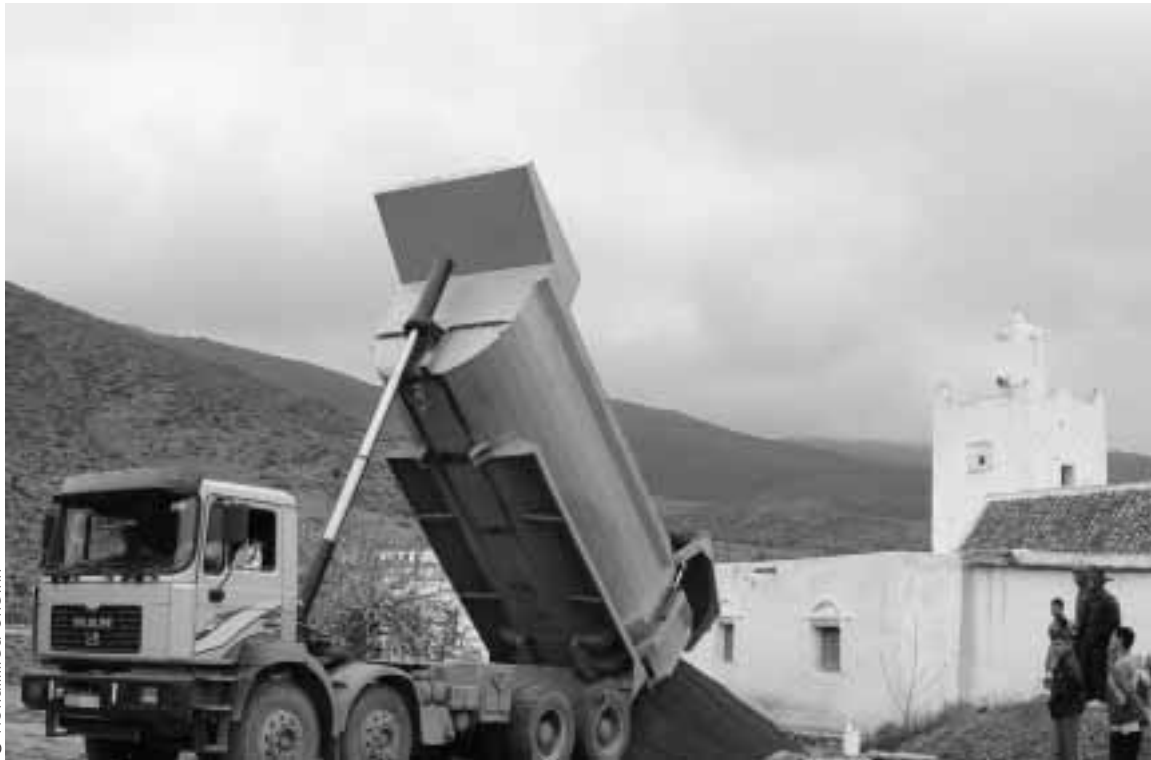
Restoring the mosque in Mestassa, Northern Morocco.
