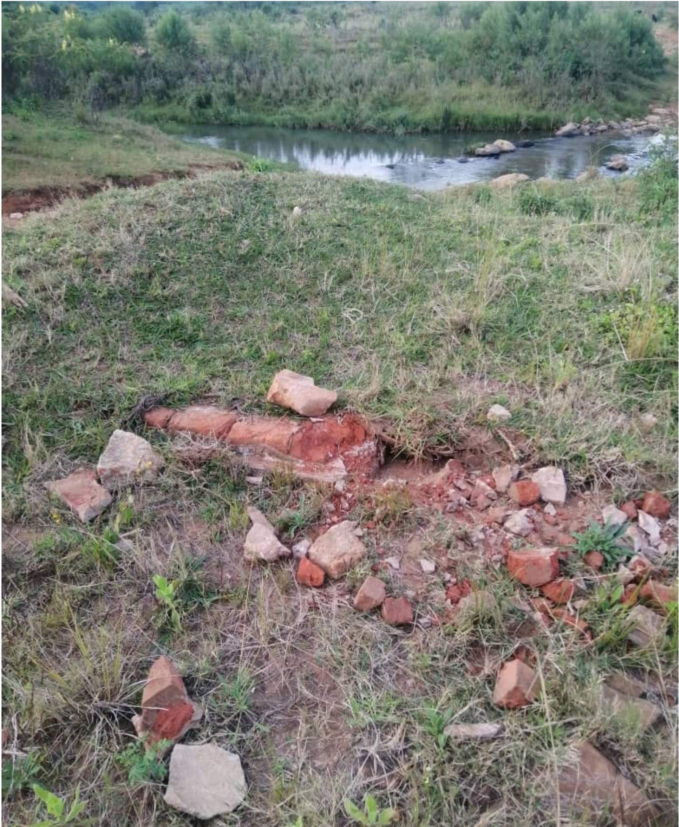
Peacock area in Chimanimani, Zimbabwe. Cyclone Idai destroyed what was once a built-up and vibrant business centre where a number of traditional ceremonies were held by the local and traditional leadership. The ICH was destroyed with the place... the bricks are what remain. Credit: Dr Lesley Macheke.
