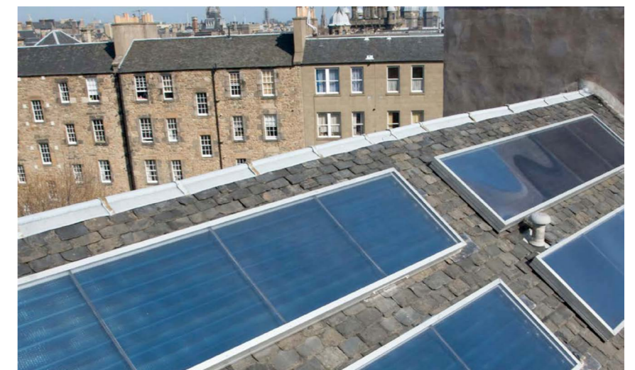
→ Solar thermal panels installed in a World Heritage site. (Historic Environment Scotland)
