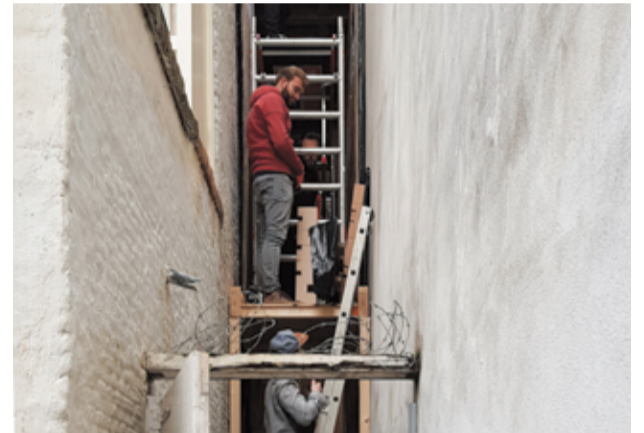
Construction process. Family, friends and local residents at work in the alley, using narrow scaffolding to assemble the Bedsteeg.
