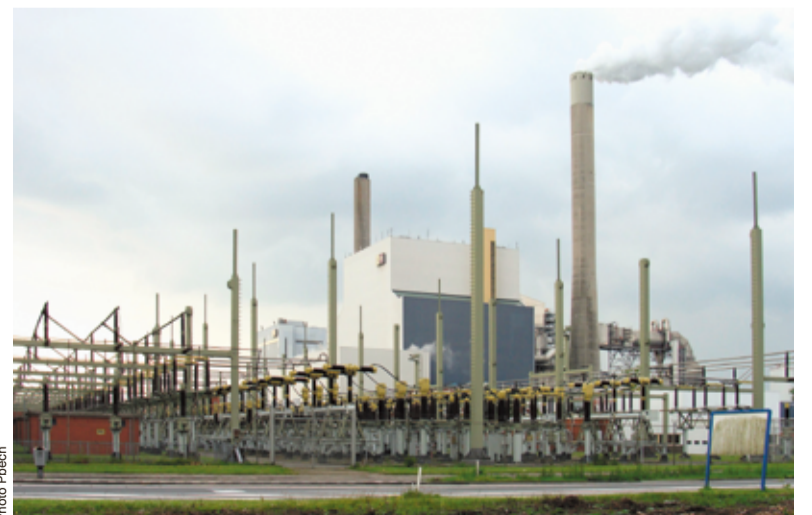
The Hemweg power plant in Amsterdam is now closed.
