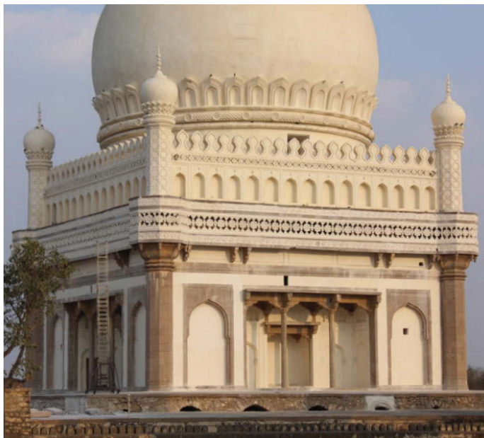
One of the ten monuments at the Quli Qutb Shah tomb complex in Hyderabad supported by the Tata Trusts, being restored by the Aga Khan Trust for Culture. Courtesy of Tata Trusts
