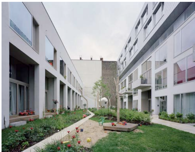
Shared space in Berlin Baugruppenprojekt BIGyard, Zelterstraße 5–11, designed by Zanderroth Architekten. Approximately forty-five kids from the families in the block can share this space, designed such that parents can share informal child-tending duties. This 1300m 2 communal yard is counterpointed by a 250 m 2 common roof terrace.
