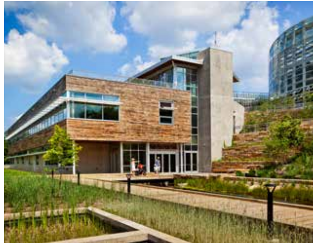
The Center for Sustainable Landscapes at the Phipps Conservatory and Botanical Gardens is designed to generate all of its own energy while treating and reusing all water captured on-site. Photo by Paul g. Wiegman.
