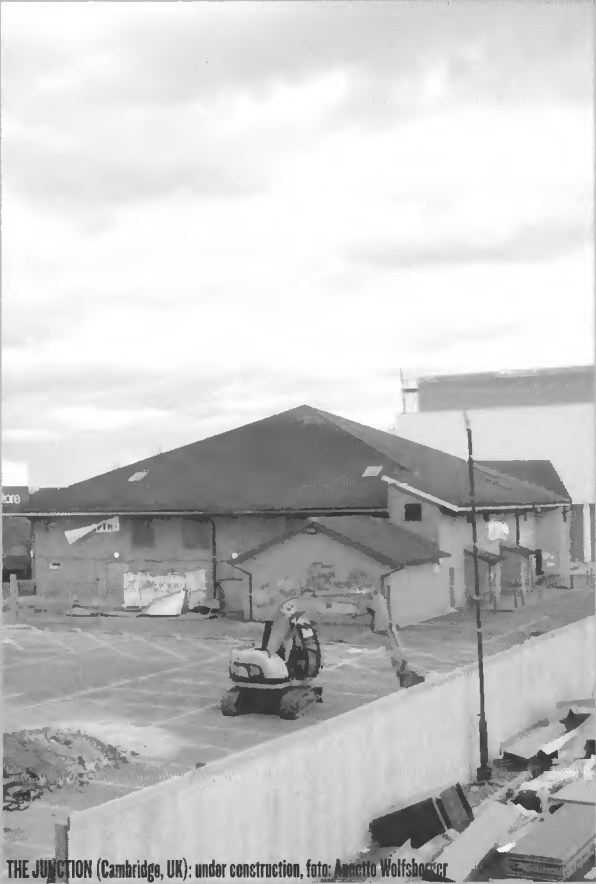
THE JUNCTION (Cambridge, UK): under construction, foto: Annetta Wolfshoer
