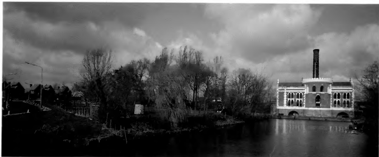
Gemaal Lijnden, one of the three pumping stations with which the Haarlemmermeer was pumped dry. The steam machines, now replaced by diesel motors, came from England, reason enough for the architect J.A. Beyerinck to use the English Gothic style for the architectural design of the pumping stations. (Archiphoto)
