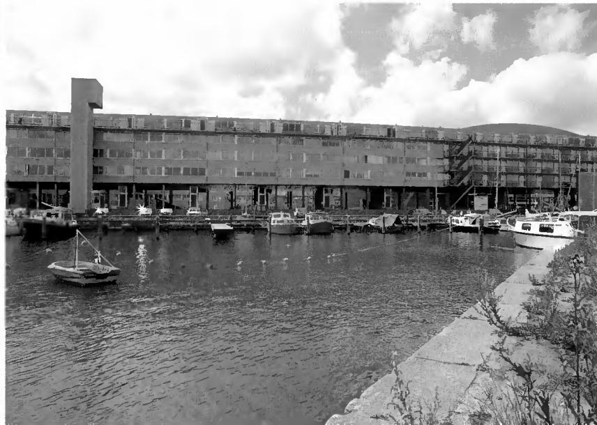
Housing on the IJ-plein. (Photos: Wim Ruigrok)
